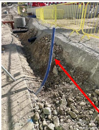
Line showing where the pipe struck the face
